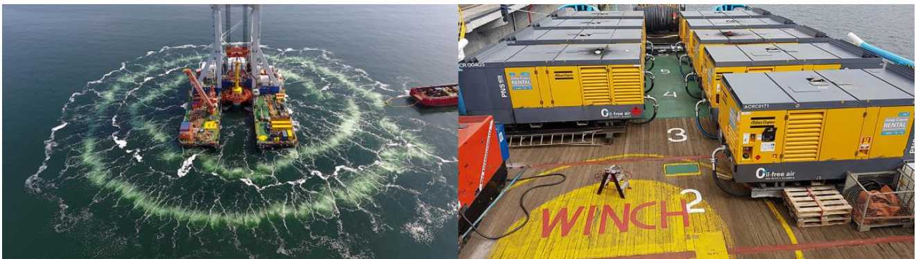
Figure 6.29: Illustration of a DBBC mitigation system (Left: in effect; Right: compressors for creating the air pressure) (Source: hydrotechnik-luebeck.de ).
